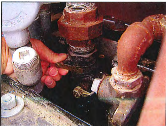
To reset the switch, first lift up the spring loaded catch.
